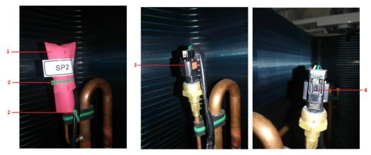
1 --- heat-shrinkable sleeve 2 --- high temperature wire tie
