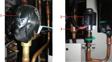
1 --- Damper block 2 --- Electronic expansion valve coil 3 --- Electronic expansion valve **Installation procedure**
