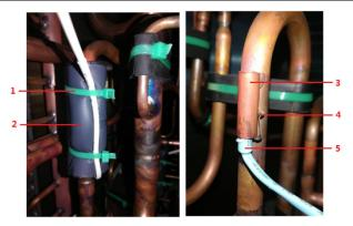
1 --- high temperature wire tie 2 --- insulation cotton 3 --- temperature sensor sleeve 4 --- temperature sensor connector 5 --- temperature sensor
